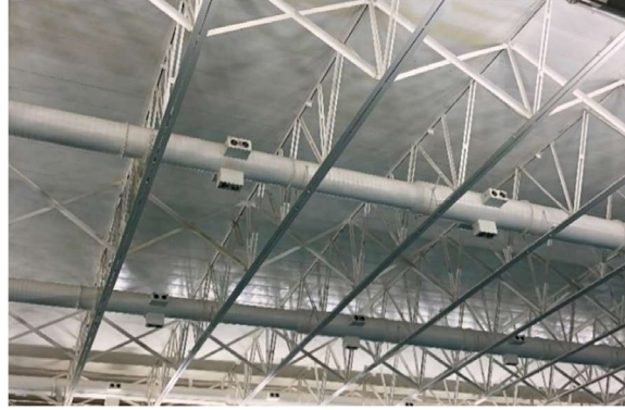
Figure 1. Open web steel joists in a roof system.
