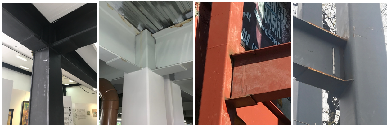
(a) With built-up box columns
