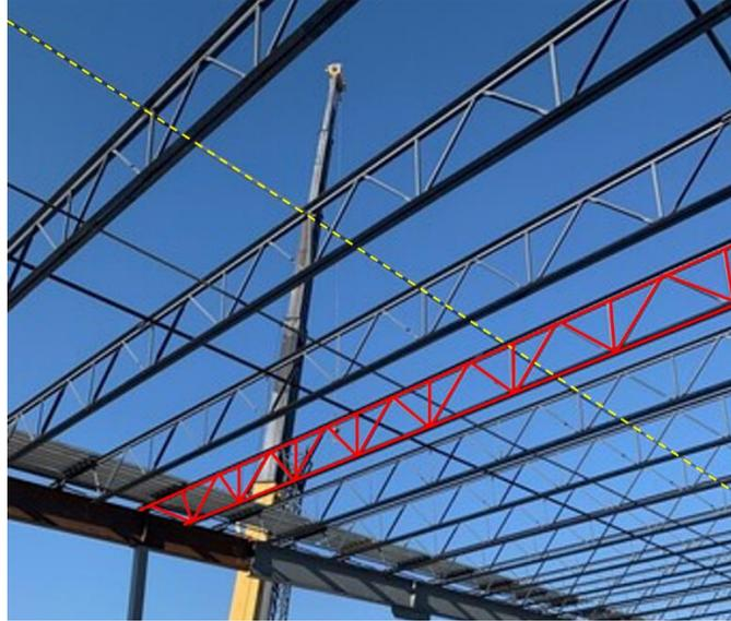
Figure 1: Roof system comprised of open web steel joists in red and horizontal bridging in yellow (SEAA 2020)
