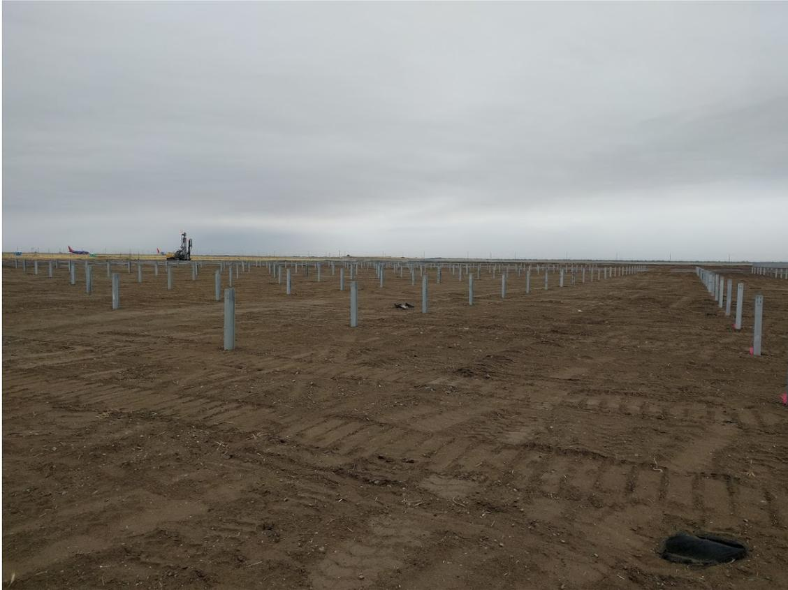
Figure 1: W-shape solar array piers
