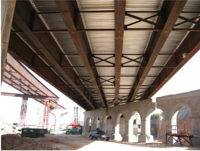
*Figure 13: Lean on Cross-Frame Bracing in Heavily Skewed Bridge.*
