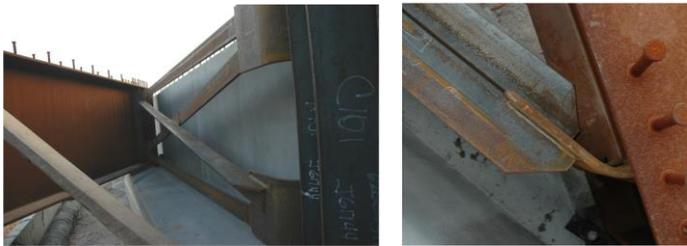
*Figure 14: Bent Plate Details Used on Heavily Skewed Bridge*
