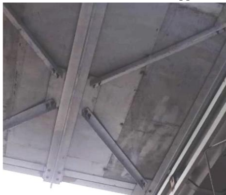
(b) Application as bracing in bridge-deck
