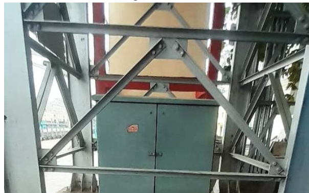
(c) Angle braces connected by two bolts
