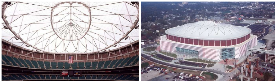
Figure 1: Real-life structural example: Georgia Dome in Atlanta. The Levy-type configuration was once the largest structural span in the world. The structure was replaced and demolished in 2015. (photo - Birdair)
